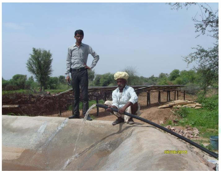
Type of pump: 4Hp 3phase Borewell Submersible Pump Total Area in acres: 10 acres Bore Depth: 4hp erected at 450ft Distance between Borewell and Solar Panel: 75m Distance between Borewell and storage tank: 10m Peak Discharge: 82LPM & 50Lpm (Low discharge models chosen due to low bore yield)
